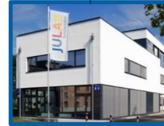
JuLab Smart building
